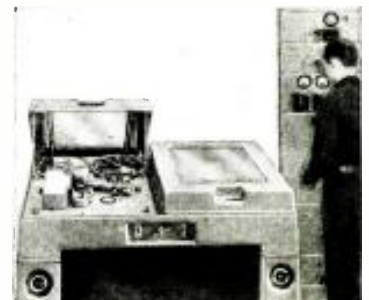
Above—PCJ's unusual sound-recording system with amplifier, etc. Left—Flat Knife Cutter which records sound tracks of varying width into moving ribbon.
