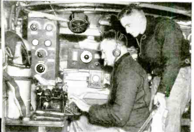
Portable short-wave transmitters and receivers mounted on motorboats and aboard trucks, so that they could move about quickly, proved extremely valuable during the flood. Above—one of the mobile units in operation at Memphis, Tennessee. This station kept in touch with the stricken areas and served as a guide for relief workers. Robert Kelly of New Orleans, La., is seen operating, while John Willmot of Mobile, Ala., looks on.
